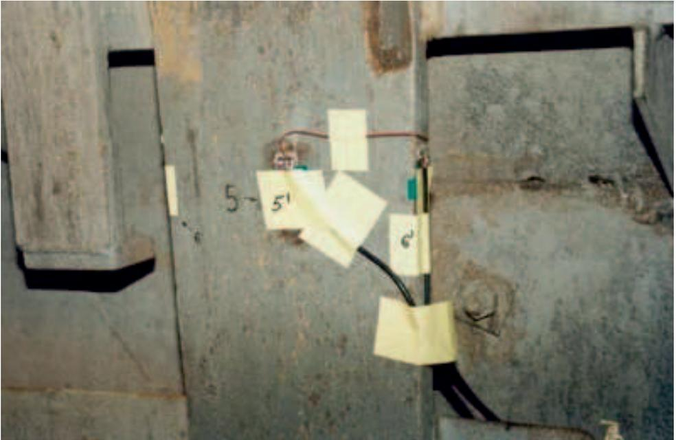
FIG. 24. Sensors TC5, TC5', TC6, TC6' fixed at the point where the mid-point string is connected with the hopper structure.
